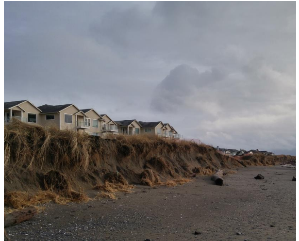
Erosion at Cohasset Beach, WA – C. Dennehy
