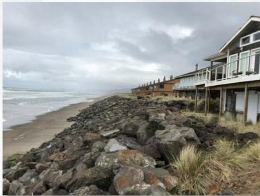
**Example Policy: Construction of riprap beach protection structures for coastal protection**
